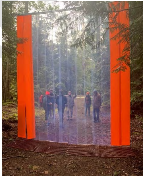
Figure 9. Examples of Freezer Curtain “doors” and Cattle Guards at Pedestrian and/or Vehicle Accesses (Tooby et al., 2022)
